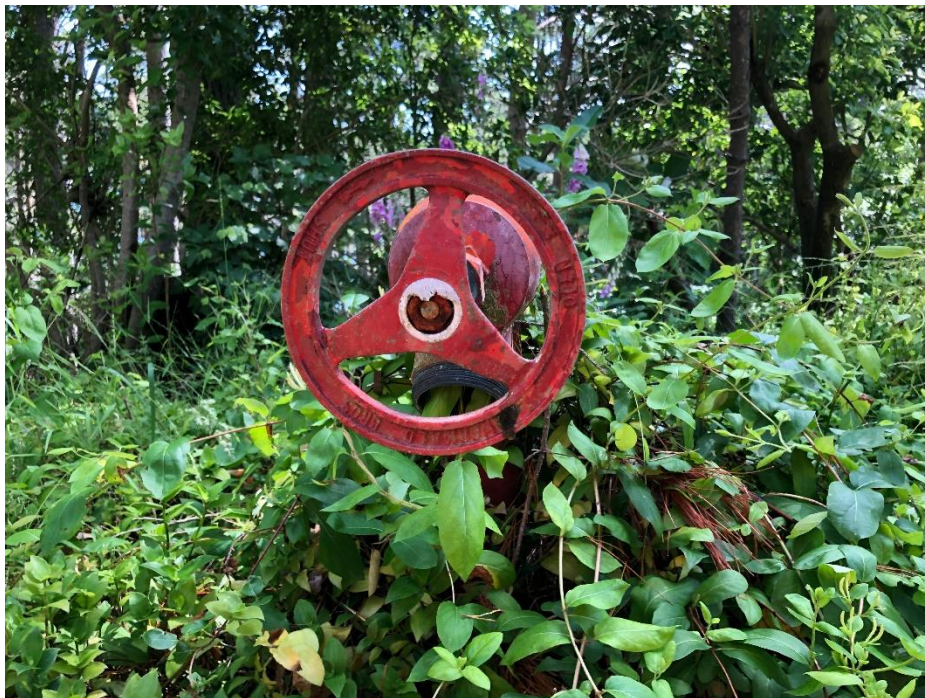
Standpipe/hydrant.
