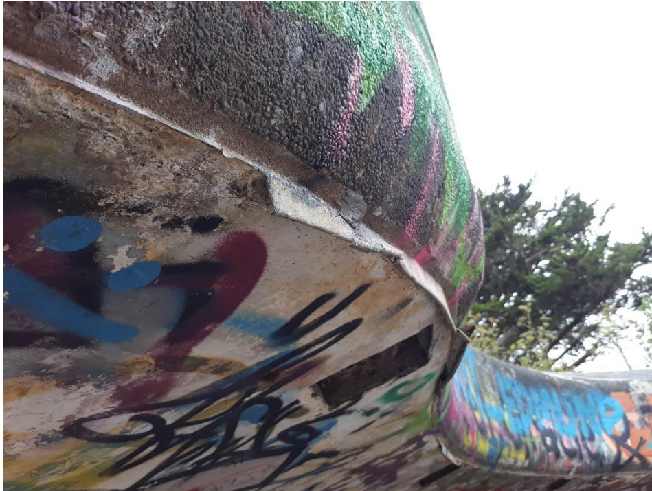
Lead flashing in sidewall to gun emplacement/battery.
