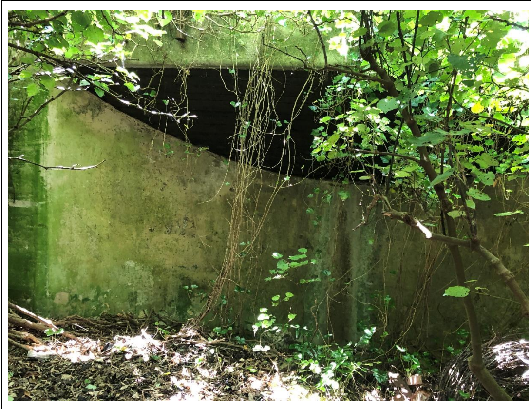
Photograph 36 Appendix B.1: Remaining structure of the 'see-saw' search light constructed of concrete and railway iron. See reel of barbed wire in bottom right corner of image
