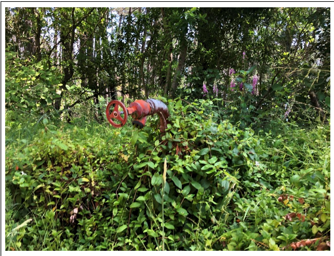
Photograph 24 Appendix B.1: Remnant valve from the former fire suppression system, visible from accessway across from Magazine E8
