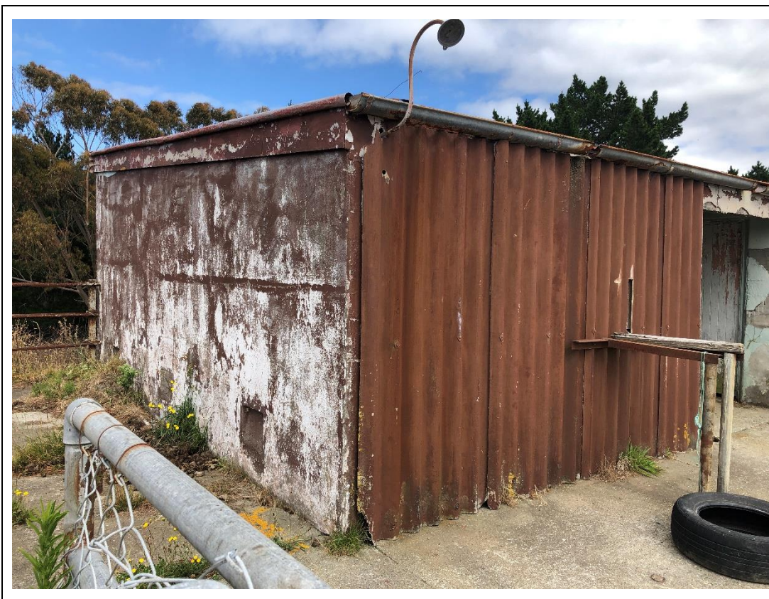
Photograph 29 Appendix B.1: Smaller farm building with Super-Six sheets on external wall and ACM sheeting on fascia
