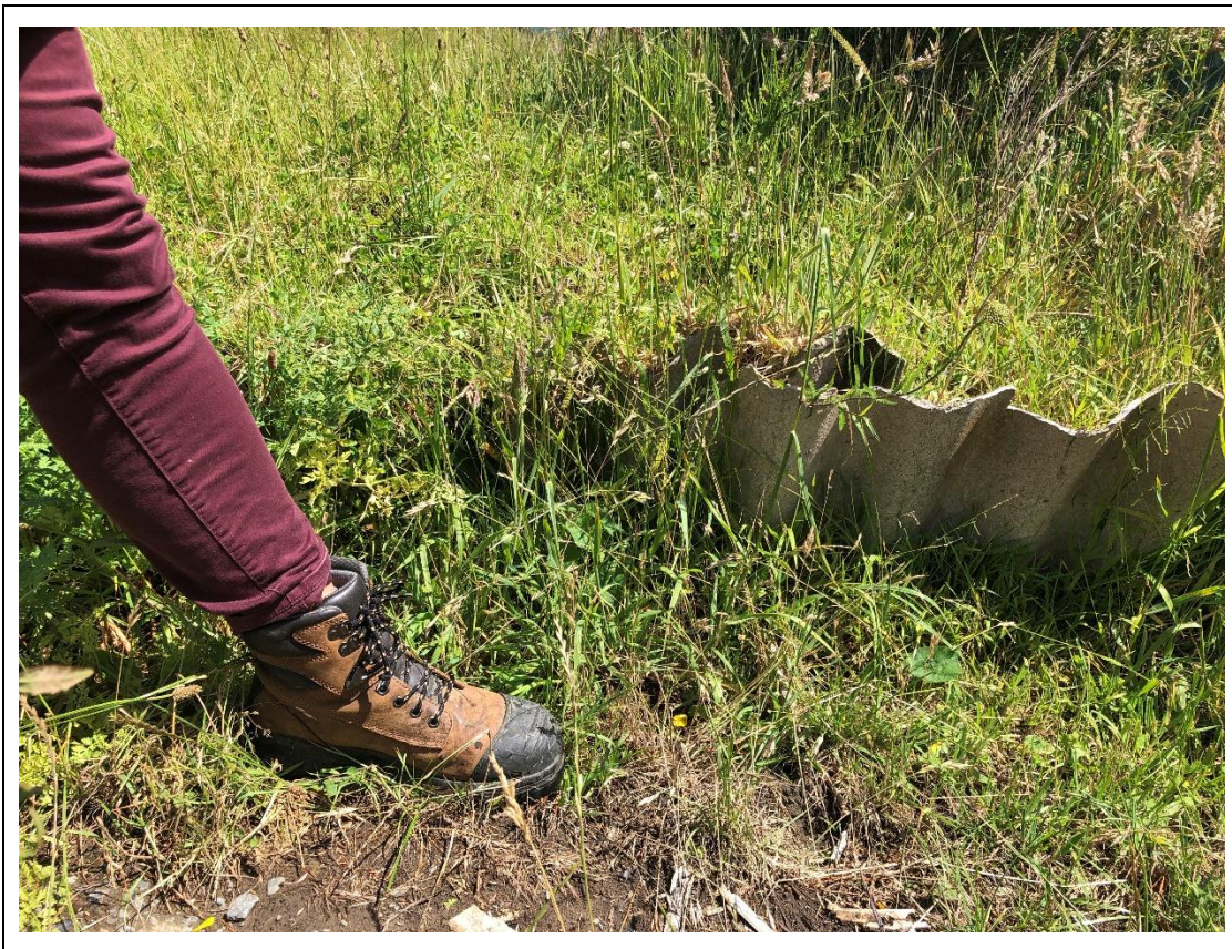
Photograph 3 Appendix B.1: Broken Super-Six sheet used as retaining wall
