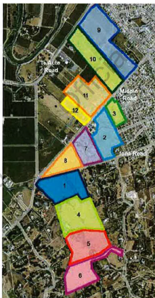
Figure 1 (Aerial photo provided by the Applicant, showing the records of title that comprise the Land) – Aerial photo of the Land
