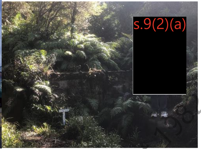
Old Railway Dam
