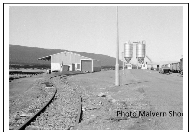
Cement silos & good shed for the Tongariro Power Scheme
