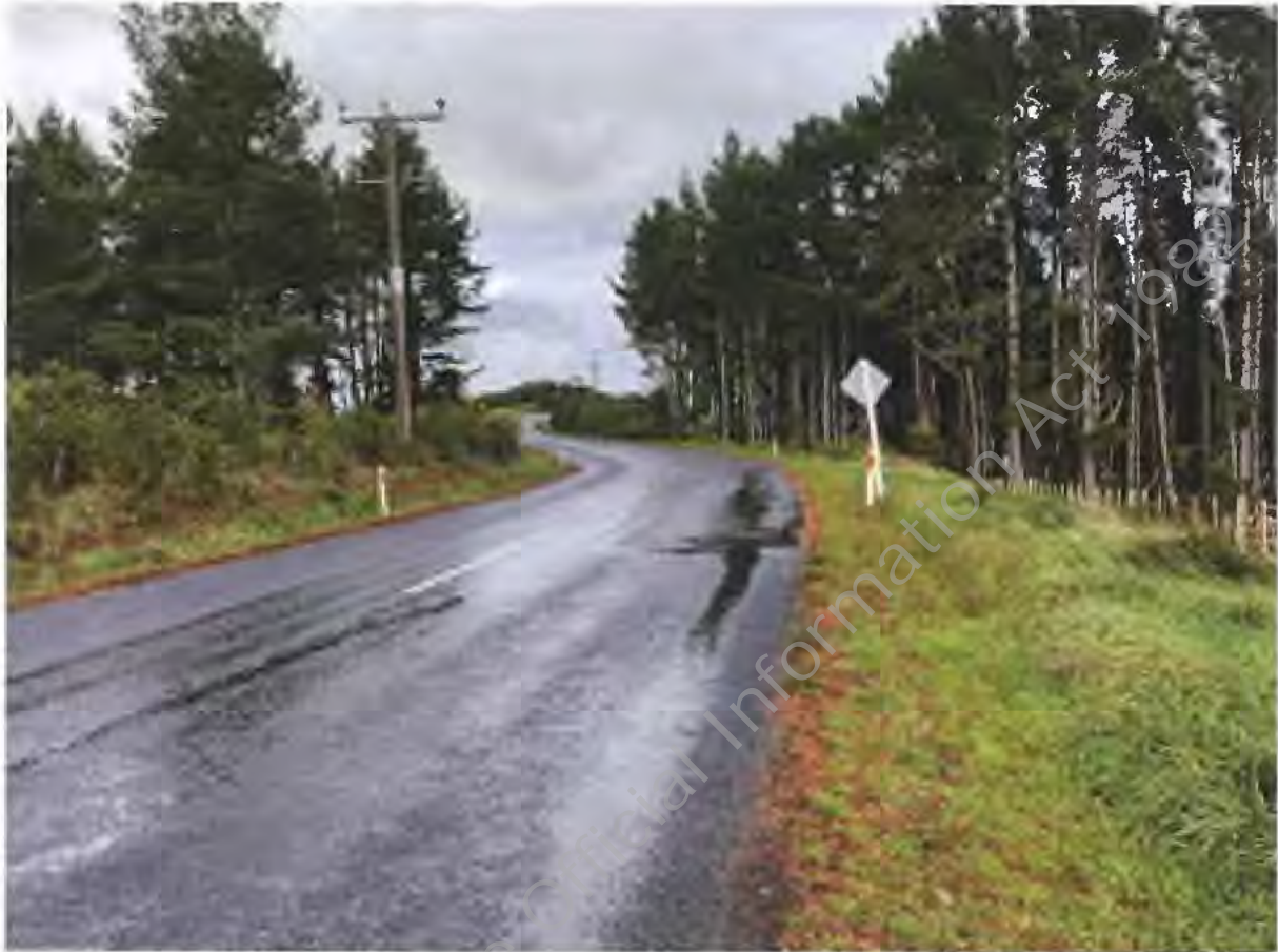
Figure 3: 537 Ridge Road Looking west
