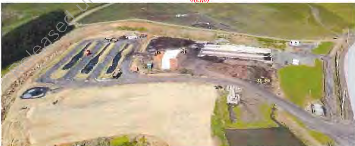
Leachate treatment plant-Hampton Downs
