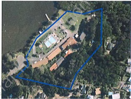
Figure 8 - Old Wharf Rd (Haruru Falls Resort)
