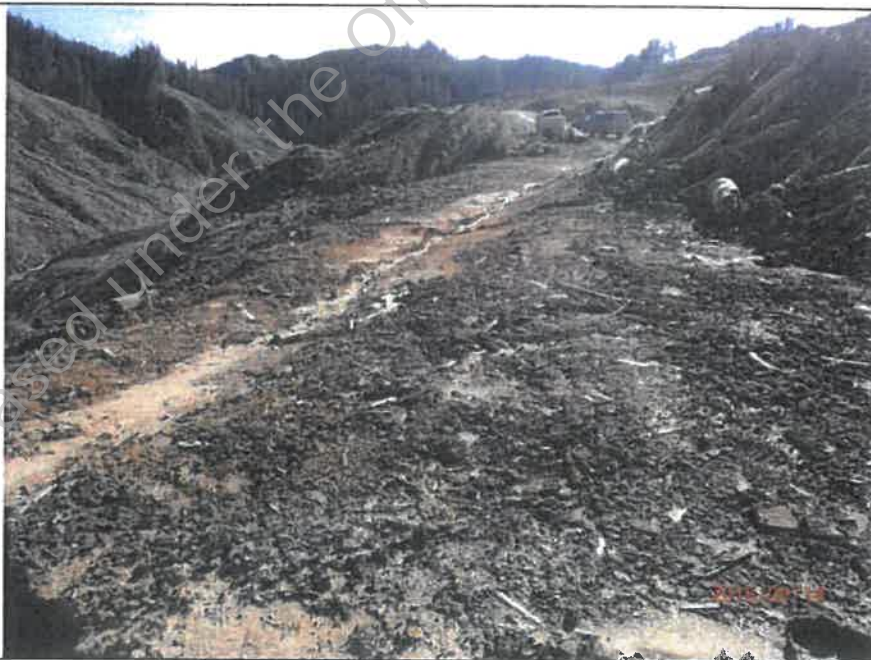
Skid site 20. Perched birds nest material has been pulled back from edge of skid and placed in stockpile. Perimeter V-drain installed to stable outlet onto ridge. Exposed ground is due for seeding by helicopter.
