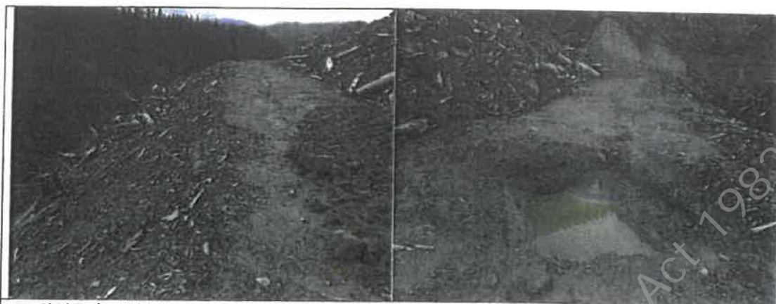
Skid 80/9 at end of Falcon Road. Logging material pulled back and stockpiled on skid. V-drain installed draining via sediment trap to slow runoff prior to discharge onto hard ground over ridge.
