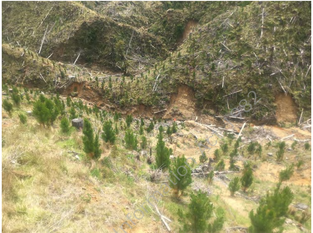
Photograph 3 below: Logging debris slide and road failure at skid 36
