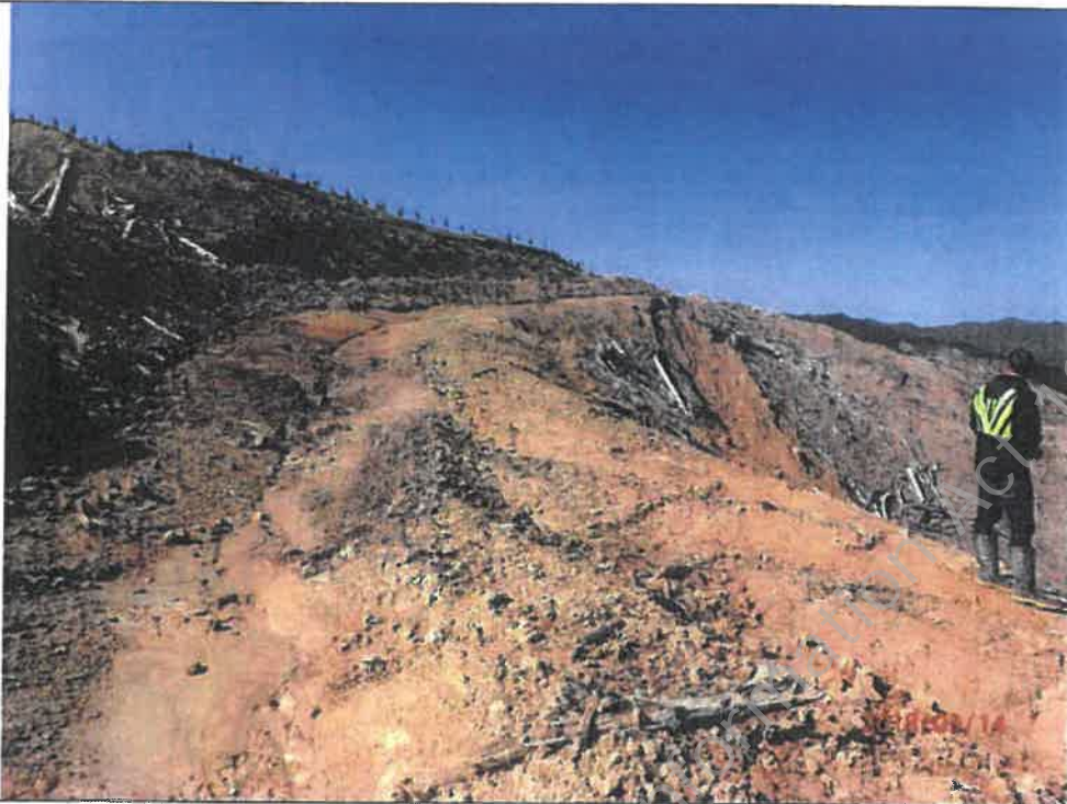
Un-named skid (Waituna Road 3.2 km). Birds nest material pulled back from edge of skid and stockpiled on skid. Perimeter V-drain installed to divert stormwater on skid to stable outlet on ridge system. Note slope of long narrow skid site.
