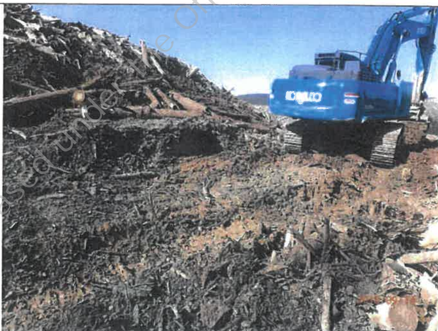
Remedial work in progress on skid site at end of Kaka Road. Very large debris stockpile and slow progress due to the type of material being shifted.
