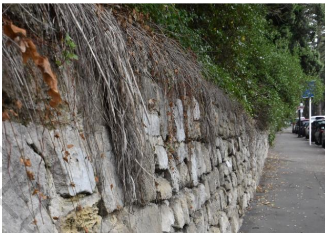
Section of squared rubble masonry, Marine Parade
