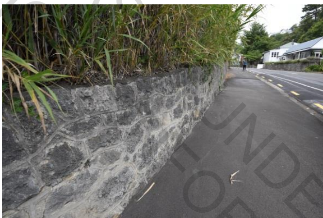
Section of random rubble masonry with repointing, Coote Road
